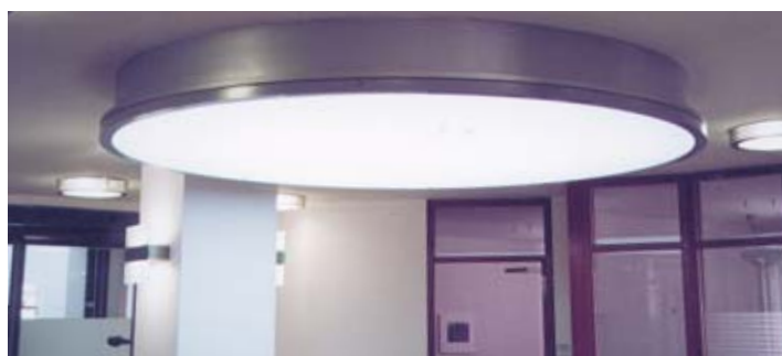
MONTAGE - Luminaire grande surface H ≤ 250 mm
